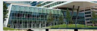
The glass surface is coated with multiple thin film layers of metal and metal oxides using the coating technology of Interpane, an advanced German company. This high performance glass has an effect of 50% energy saving in comparison to that of general glasses and of anti-condensation.
